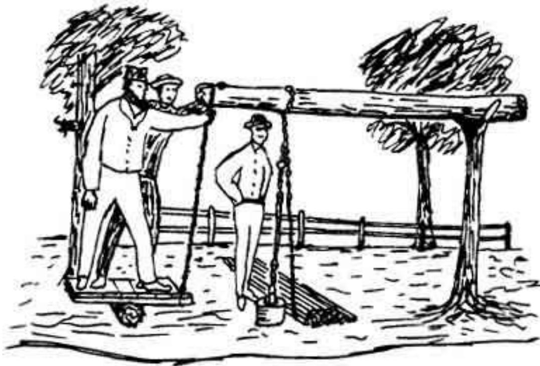
The anchored butt end of the spring-pole would be off the drawing to the right. The connecting rope for the teeter board in this example is tied at the working end of the spring-pole instead of behind the tool string. Drilling rods are piled on the ground ready for use. The number of them suggest that this well is programmed to eventually reach close to two hundred feet. This drawing is derived from a drawing believed to represent an early 1800's drilling method.
