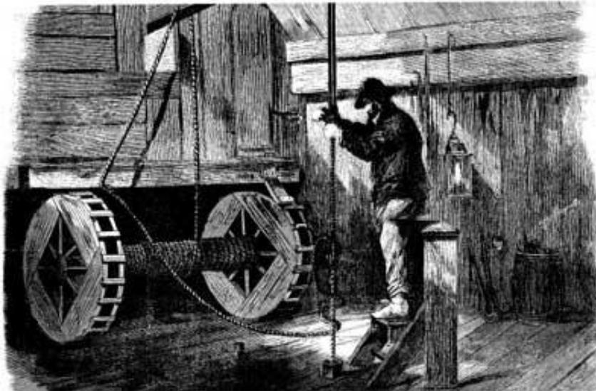
One of a pair of treadle rim bull wheels lies in the left foreground in this Mather photo of the 1862 Sherman Well in Oil Creek Valley. The round shaft is clearly visible, but the wheel that would have been on the right end of the shaft is missing. The remaining wheel served as one of two circular treadles operated by foot power and used to take up drilling rope and spool it on the shaft.
