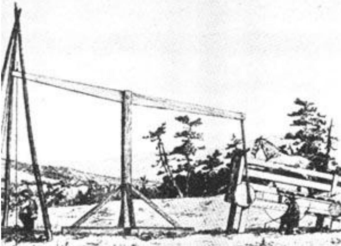
A walking horse, doomed to spend its shift trodding but going nowhere, provided power. The treadmill ran like an exercise machine. A horse and treadle arrangement served to operate a walking beam rig and could have done the same with a spring-pole. It was a matter of hooking it up right. This means of drilling goes back to the salt days and, after a fashion, even before then.
